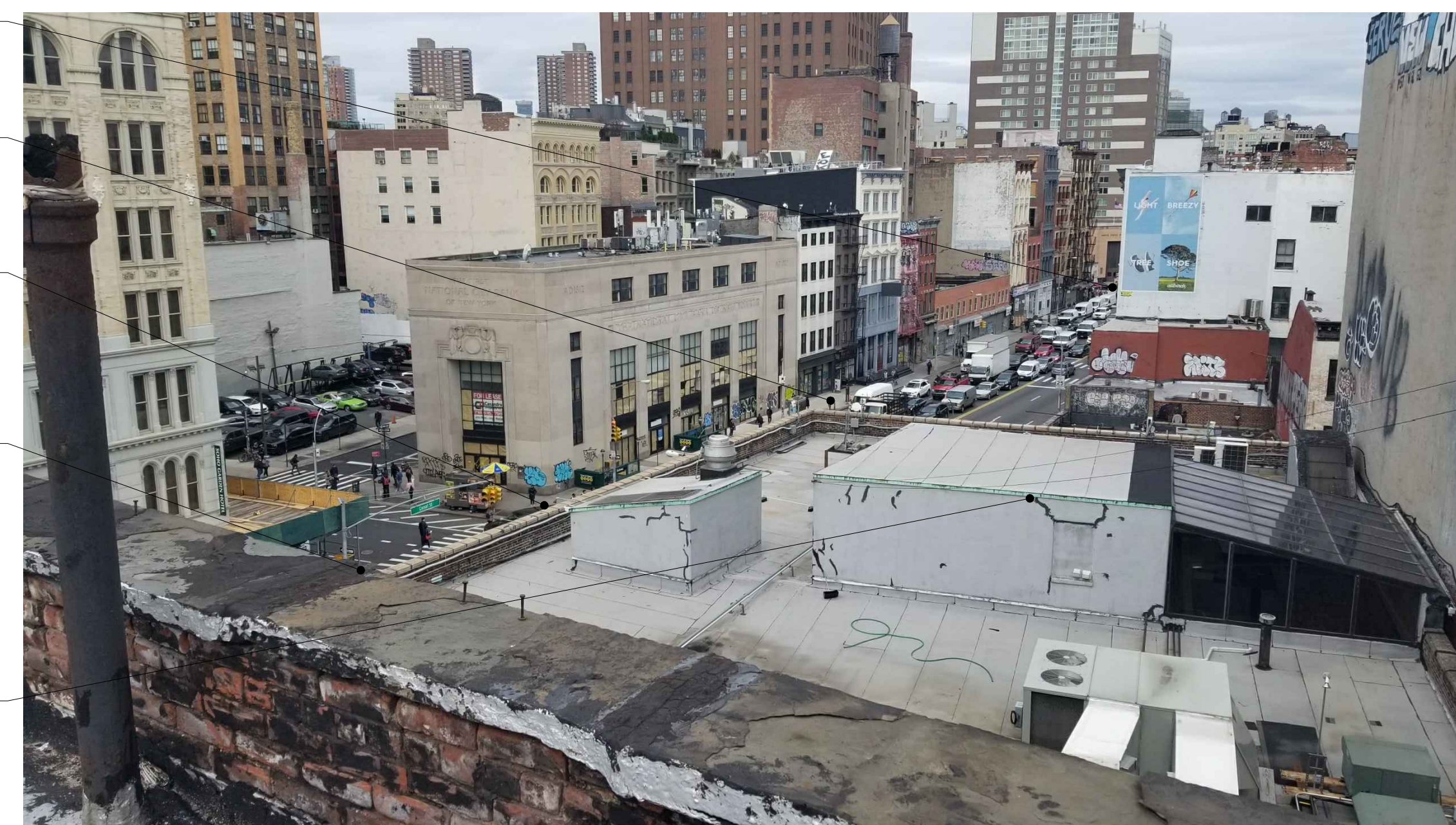
VIEW FROM 275 CANAL ROOF AT APPROX. LOCATION OF UNITS
