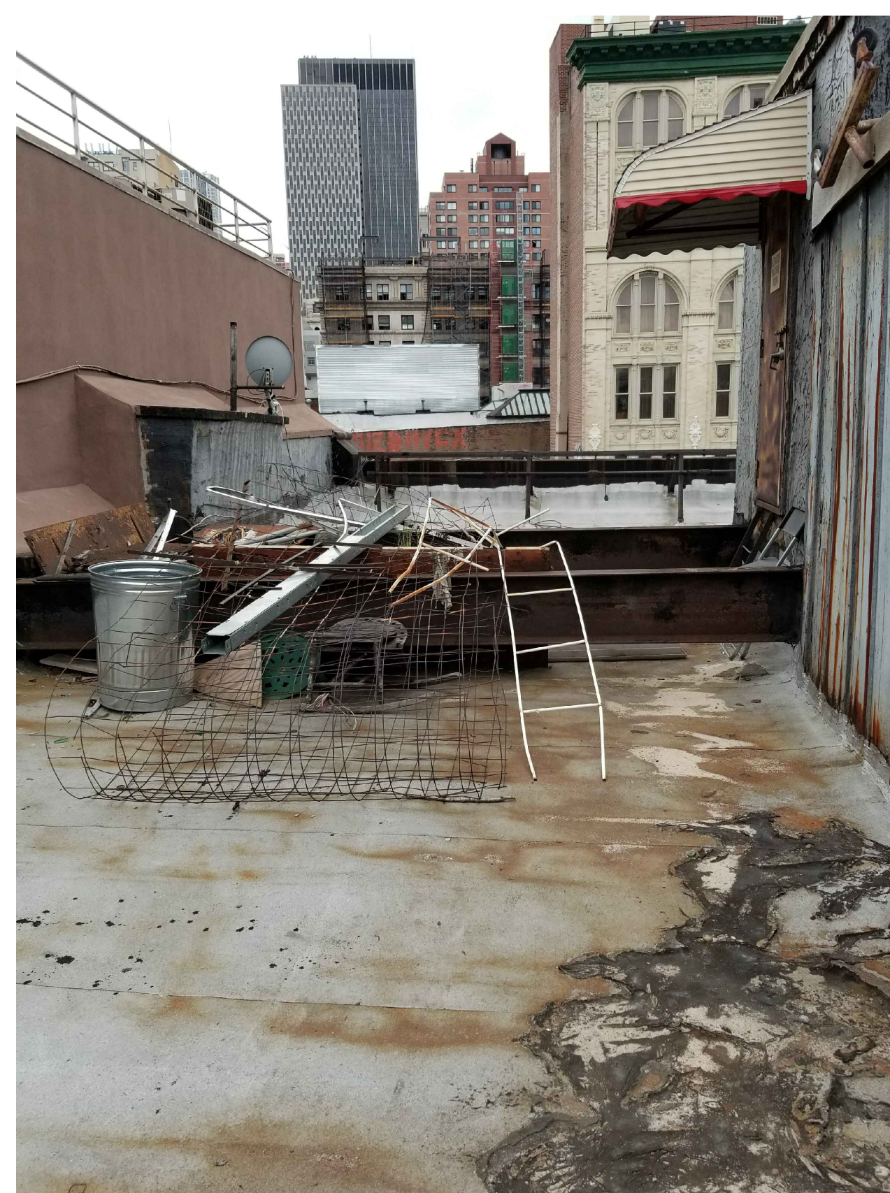
02 EXISTING ROOF — FACING SOUTH NTS
