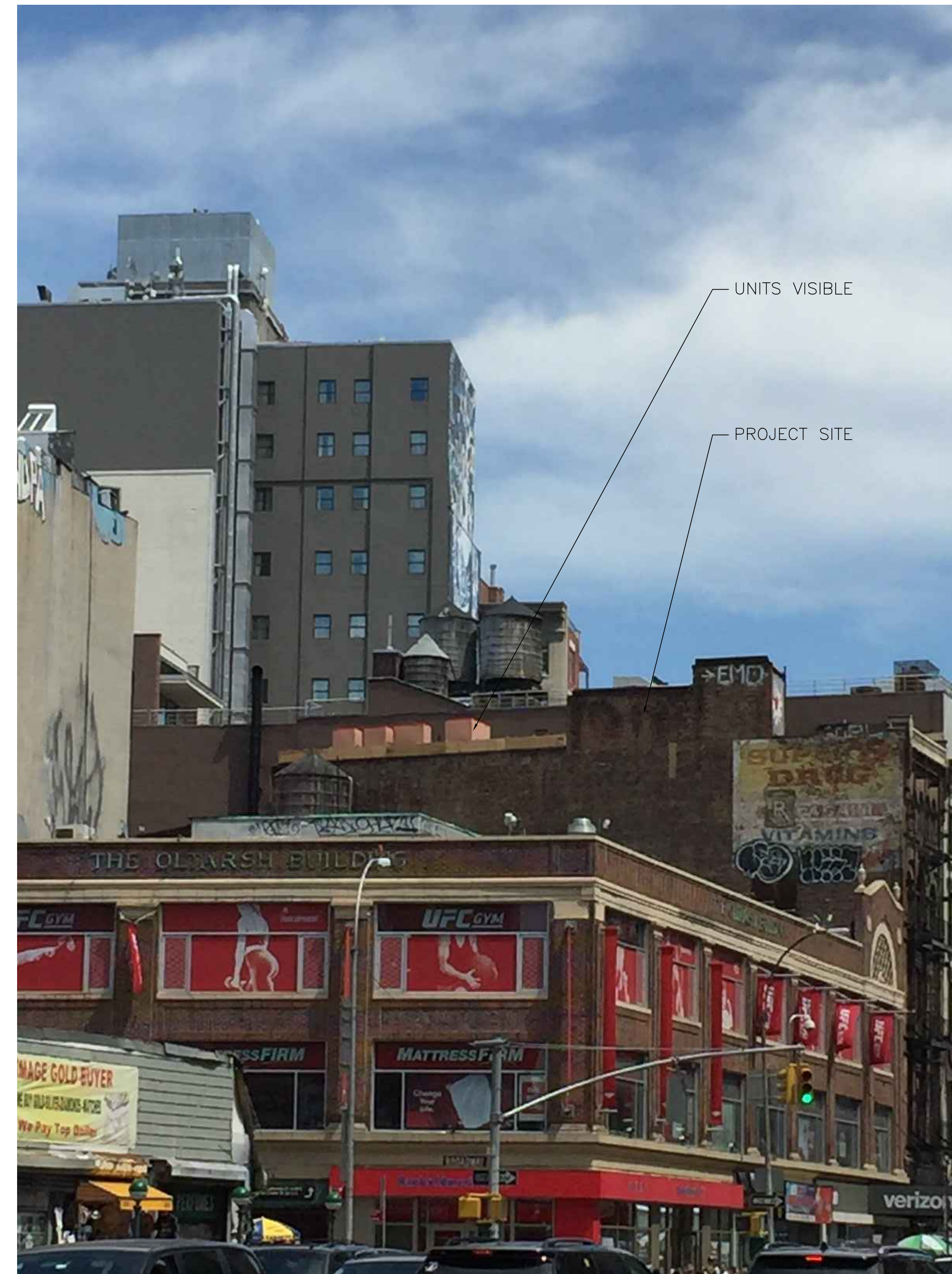
B ZOOMED IN VIEW ACROSS FROM CORNER OF MERCER ST AND CANAL ST (UNITS VISIBLE)
