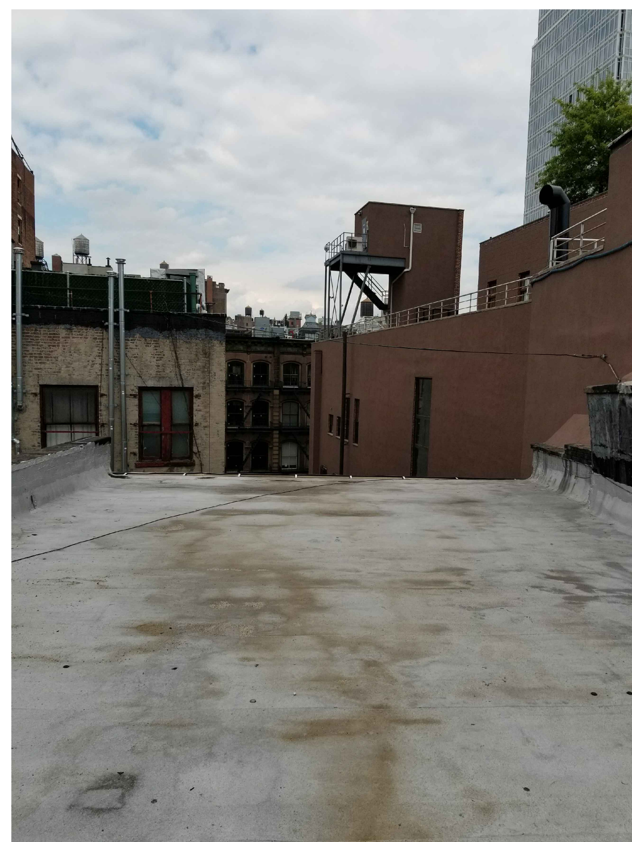
01 EXISTING ROOF — FACING NORTH NTS
